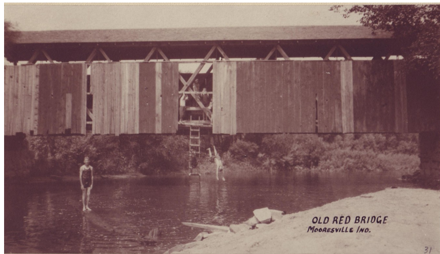
Old Red Covered Bridge on Waverly Road, Mooresville, Indiana (Early 1900s-1910s)
