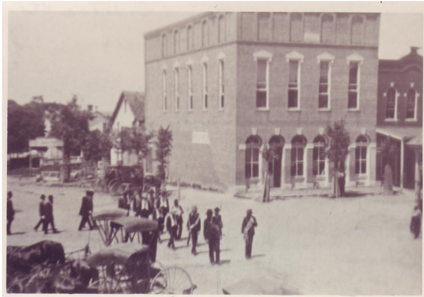
Second I.O.O.F. Building, Downtown Mooresville, Indiana (1881 to mid-1960s) (Circa 1885 Photo)
