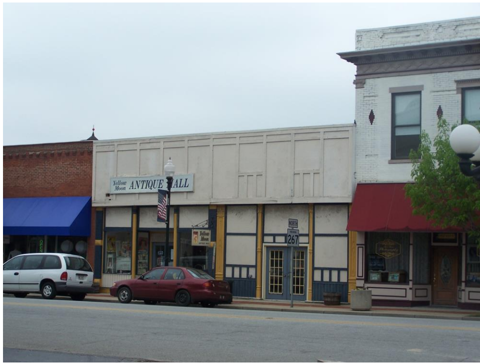
Figures 18A & 18B. The north side of West Main Street (May, 2008), showing (above, left to right) the old Carnegie Library, 12 (and part of 10) West Main Street; and (below, L to R) part of 12, and 10-8-6 West Main Street.
