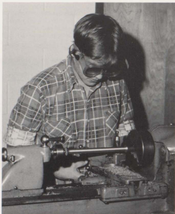
Junior Gary McKinney operates the lathing machine to achieve a pre-determined size sheet of metal.
