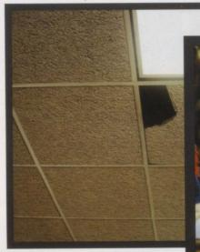
Some of the ceiling tiles were broken and leaked water.
