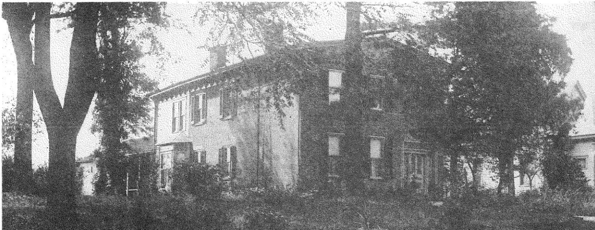
Figure 2. The Conduitt-Moore house at 35 West High Street, which is the only Moore home still standing today.
