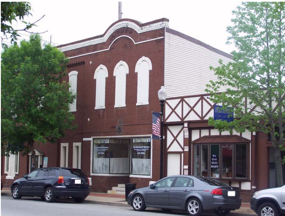
Figure 7. 20-18-16 South Indiana Street (May 2008).
