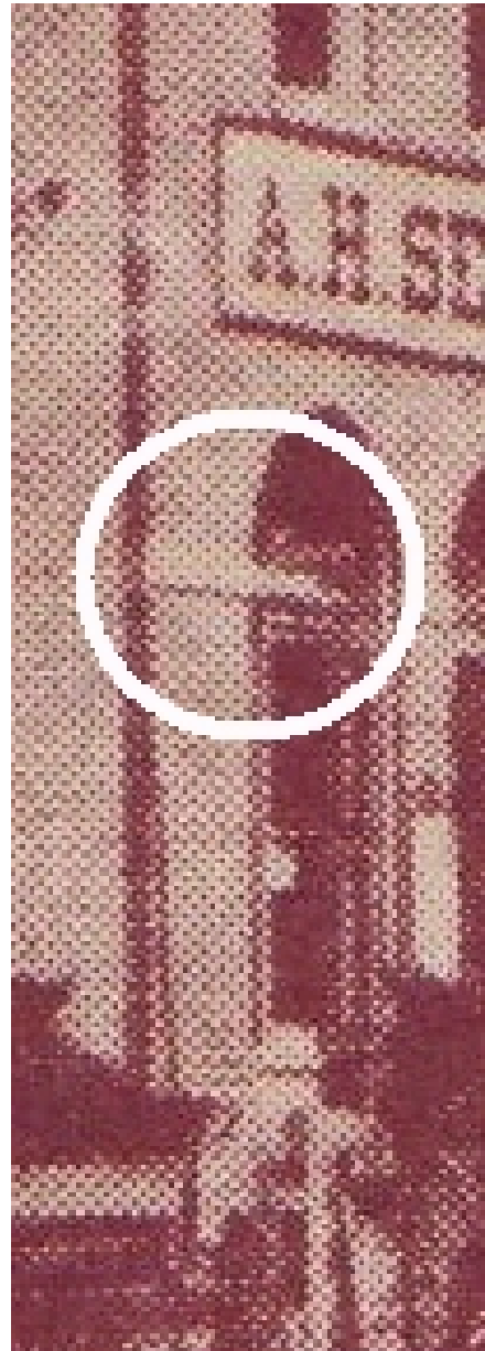
Figures 3C & 3D. Notice the concrete lintel running horizontally from the windows to the brick setback, which matches in both pictures
