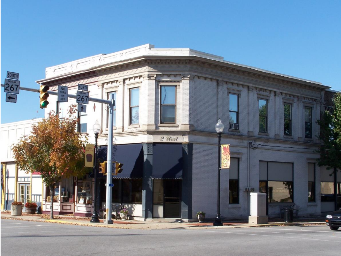
Figure 14. The northwest corner of the intersection of Main and Indiana Streets (Oct. 2007), showing the former location of Farmers State Bank. Roscoe Stovall, Jr. & Associates, attorneys at law, currently conduct business at this location.
