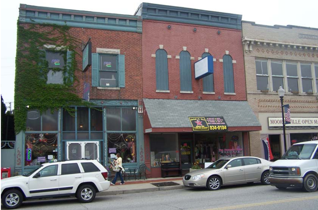
Figure 6. Buildings at 11 (left, now Zydeco's 5 Restaurant) & 9 (center, now Spotlight on Stars Dance & Tumbling Academy) East Main Street in May, 2008. The Keller
