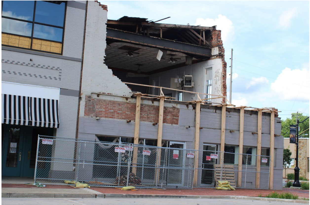
Structural Support to the Bass Building (July 2020) (photograph by William R. Buckley)
